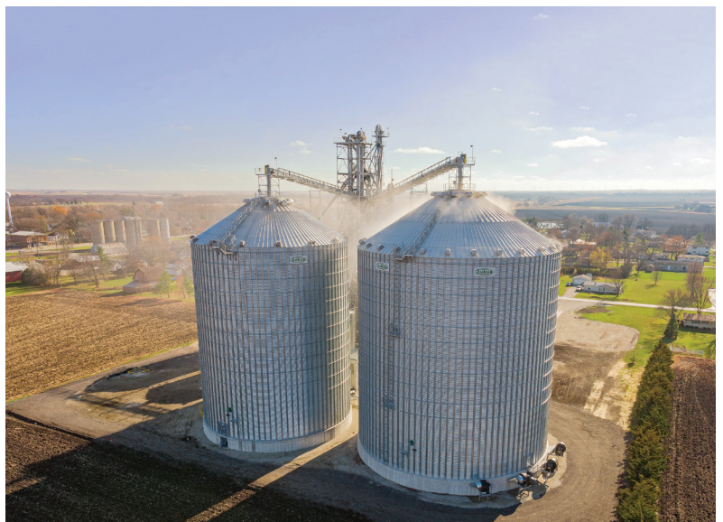
*Standard roof peak loads meet ASCE 7-10 for unbalanced snow load with 40 psf ground snow load.
