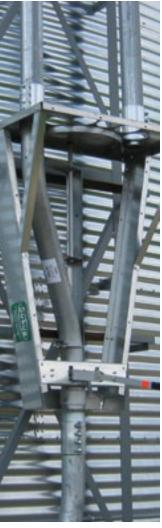
7-Way Distributor Valve routes grain up to seven bins quickly and easily. Can be mounted horizontally or vertically. When mounted vertically, the valve is operated from the bottom.
